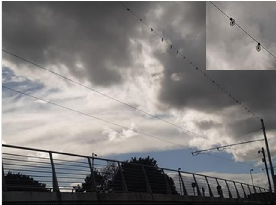
Figure 2-1 Bird deflector/ flight diverters on the Anne Devlin Luas Bridge, Dublin.
